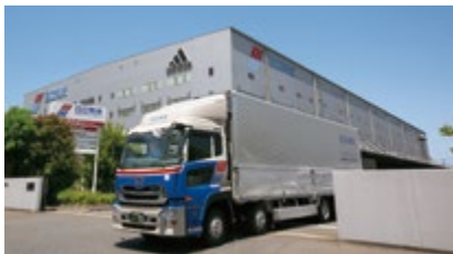
Hitachi Transport System's Metropolitan East Distribution Center and a large truck.
