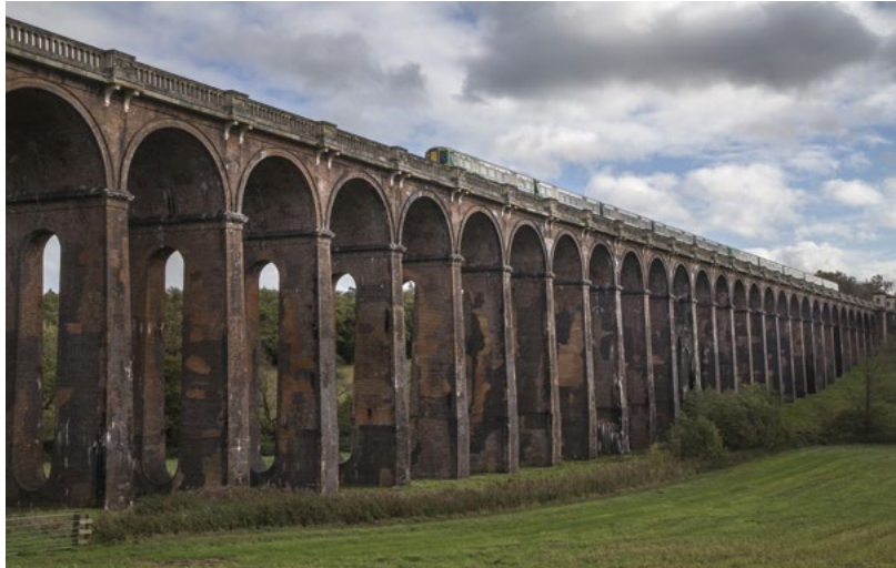
The London–Brighton rail line runs atop England's Balcombe Viaduct, completed in 1841.
