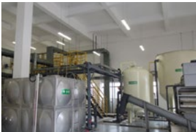
A wastewater treatment facility.
