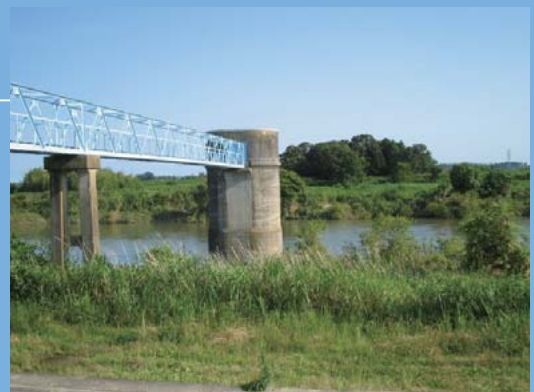
Kujigawa River Water Tower today
