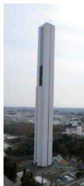
New elevator research tower at the Mito Building Systems Division of Hitachi's Urban Planning and Development Systems Company
