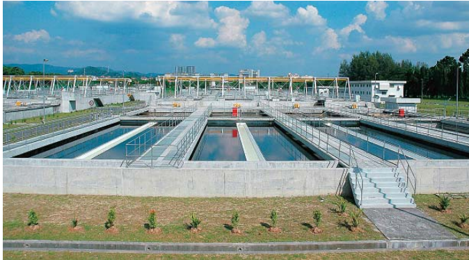
Bunus sewage treatment plant in Malaysia
