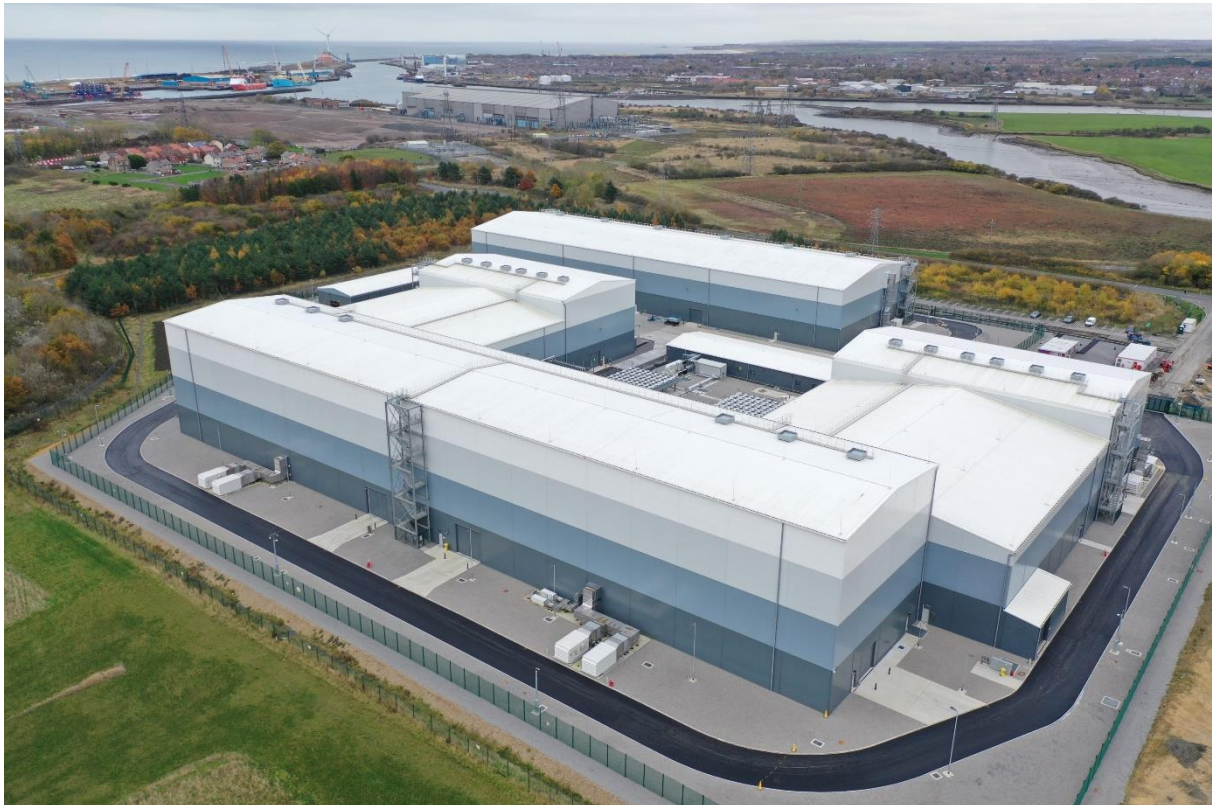
North Sea Link – Blyth Station in the UK
