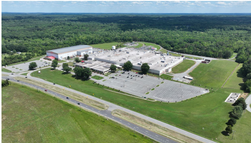
Hitachi Energy's South Boston manufacturing facility
