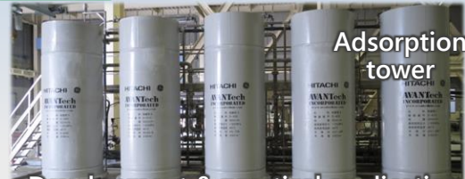
Adsorption tower Development & practical application Of simultaneous adsorbent for radioactive cesium and strontium
