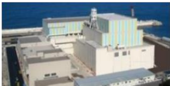
Nuclear Power Plant (ABWR)
