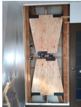
Column-mounted anti-seismic oil damper system
