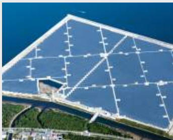
Photovoltaic power generation systems (Mega solar)
