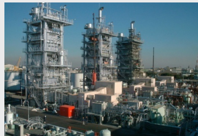
Power generation business
