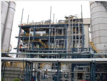
High-functional plastics production facility
