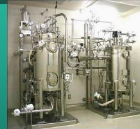
Biopharmaceutical manufacturing plant
