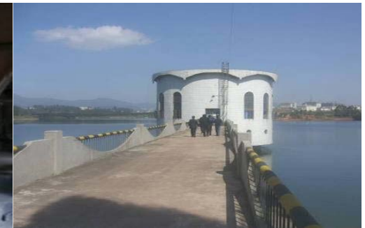
(For intake pump)
