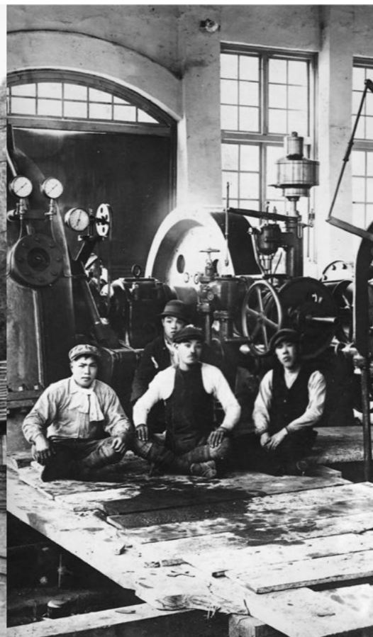
The power station at the Hitachi mine (1916)
